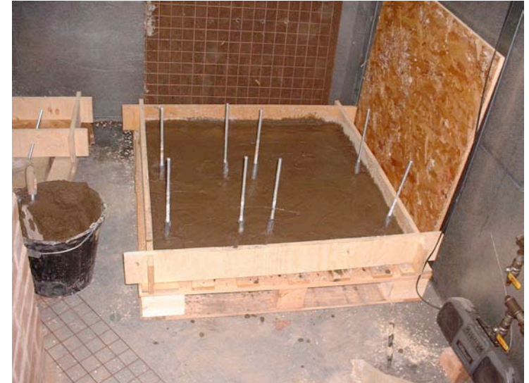
Photo 4: ... former side plates with ... cement and screwed rods
