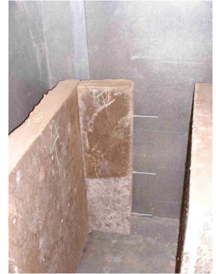
Photo 6: Fitting rear panel first before centre and front panels
