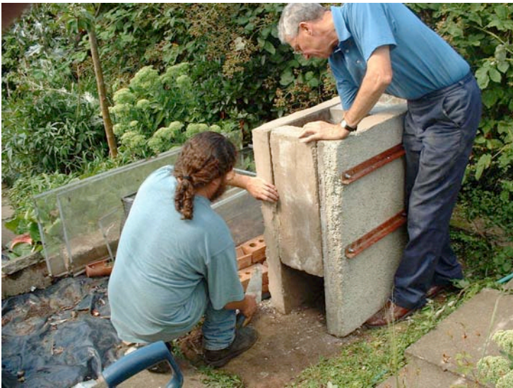
2. Sides are assembled and gaps filled with fire cement
