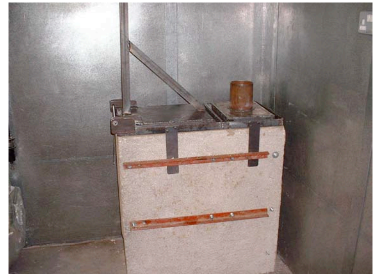
Photo 9: Fitting steel top
