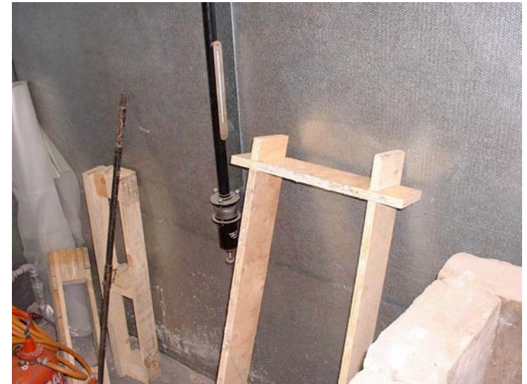
Photo 2: Cement former assembled for front and centre cross-pieces
