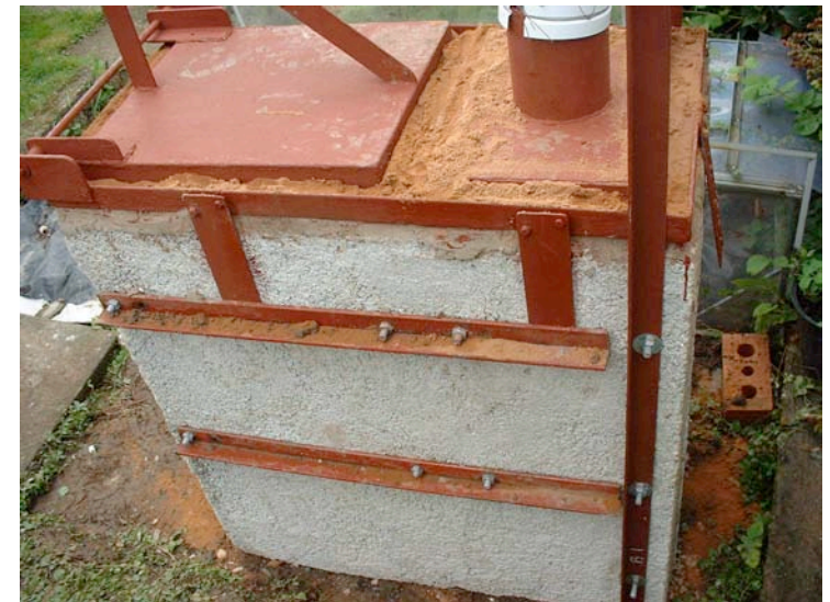
4. Incinerator complete and operational. Chimney support brackets attached and chimney erected
