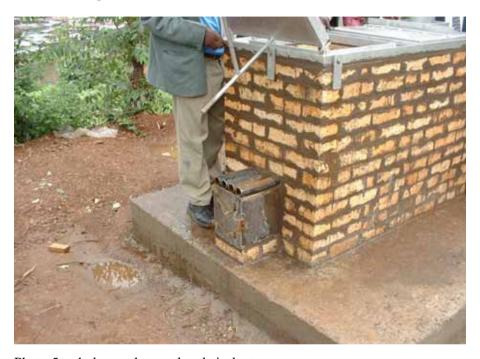
Photo 5: ash door, ash tunnel and air ducts
