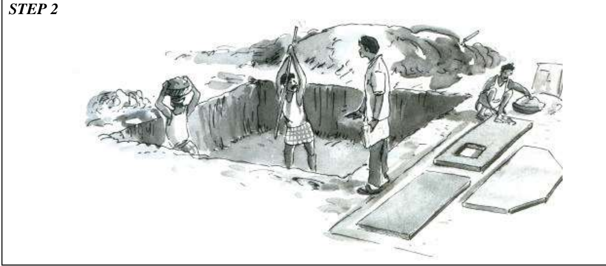
Figure 2.3.2 Digging WDU foundation and ash pit
